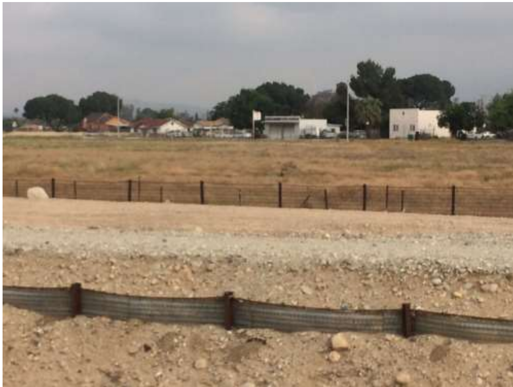
Photo 1. Facing north toward 5 th Street at vacant field adjacent to the City Creek Bypass Channel. An example of the BUOW survey area.
